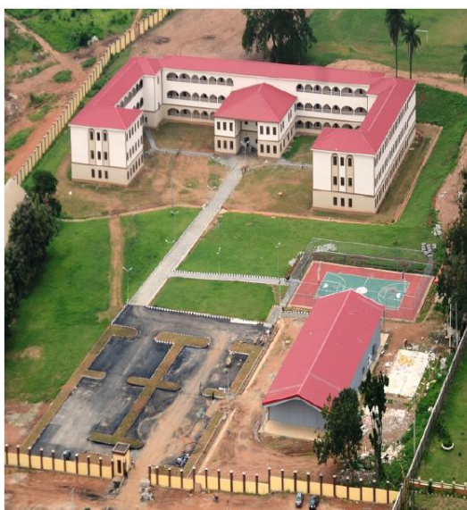
Plate 8: One of the mega schools constructed by the state government.
