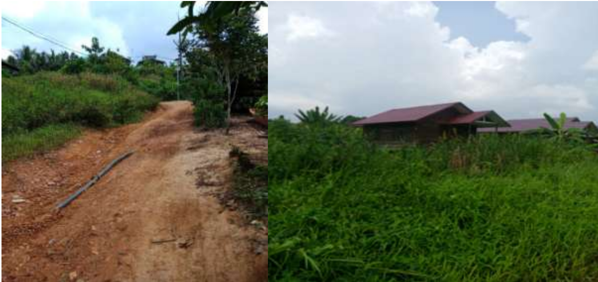
Access road built by PT.KPC
